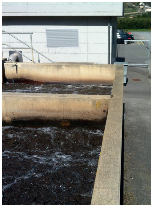
Above: Uncovered bioreactors at Saillon in Switzerland were the source of the biomedia lost to the environment © Surfrider Léman
