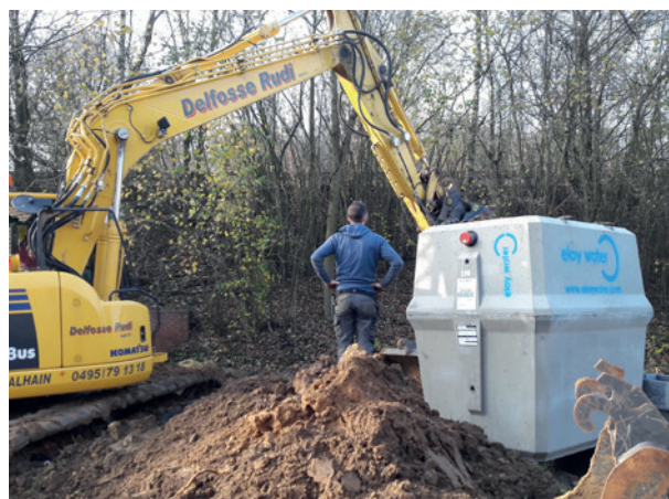
Above: Installation of a micro purification Oxyfix® plant ©Eloy Water ( www.eloywater.fr )
