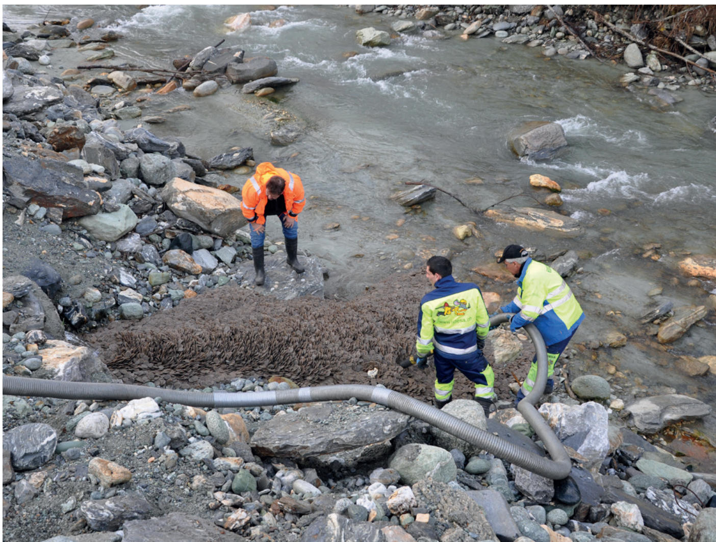
Above: Attempts to recover biomedia lost from the wastewater treatment plant at Evolène © Frank Odenthal
