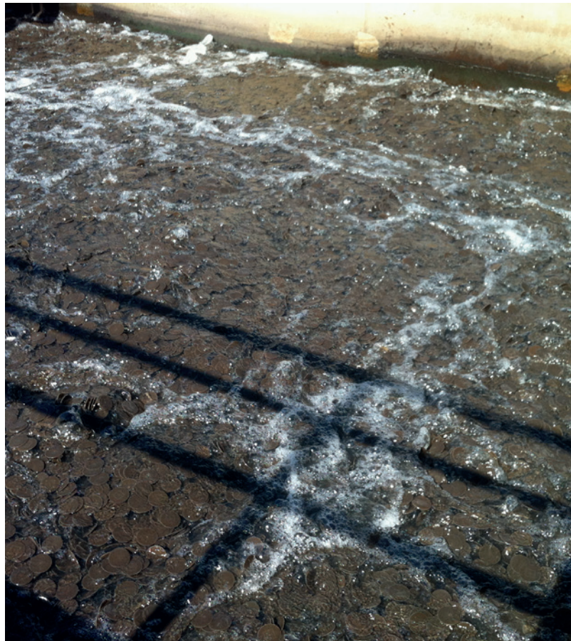
Above: Moving bed bioreactor at the WWTP in Saillon (Switzerland) © Gaël Bost / Surfrider Léman
