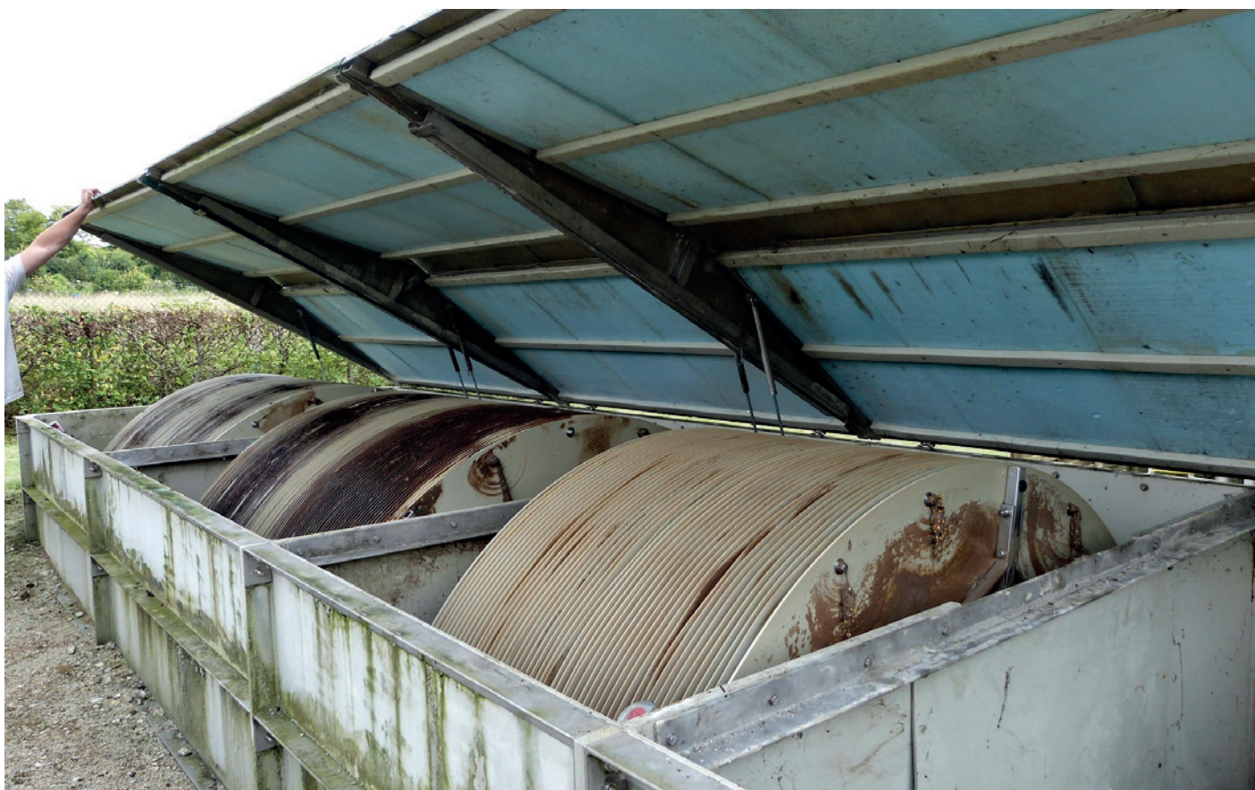
Above: Rotating biological contactors © Roinville-sous-Auneau city
